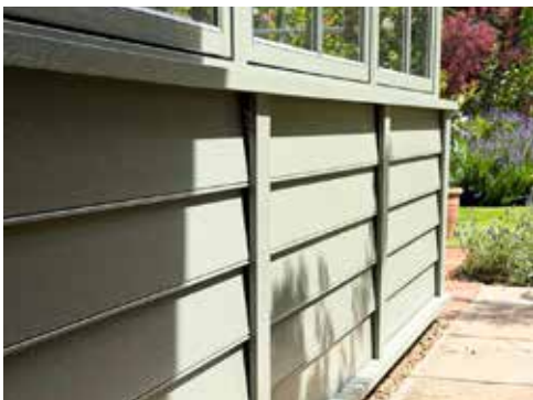
Greenhouse with timber panelled base
